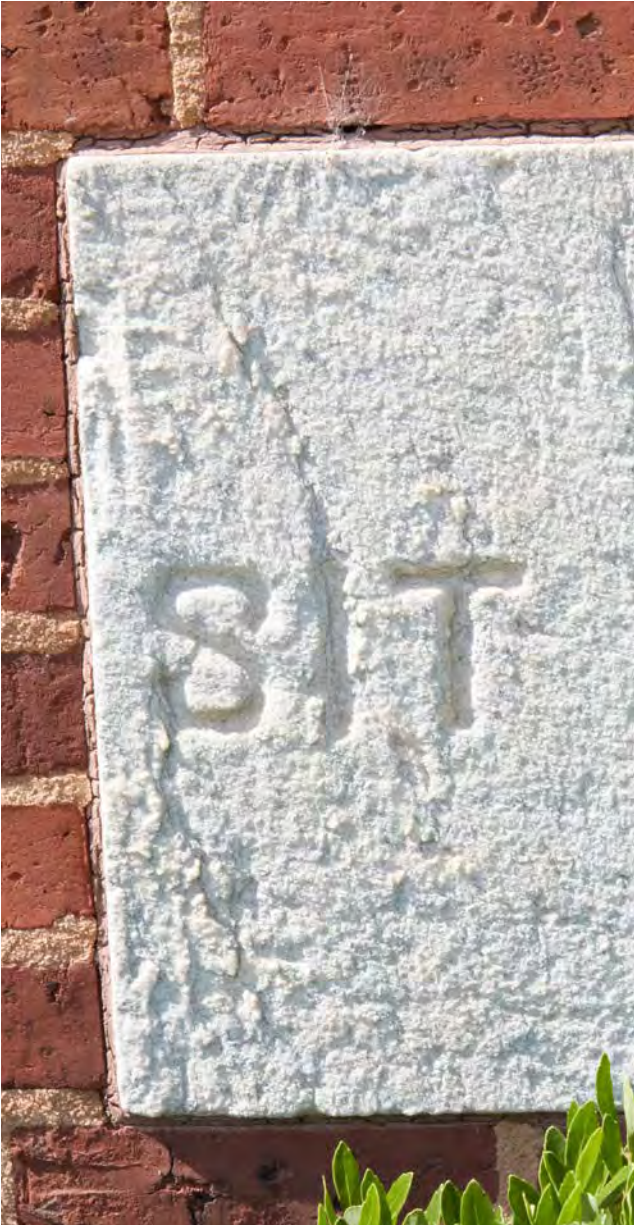
Embedded within the foundation of His
